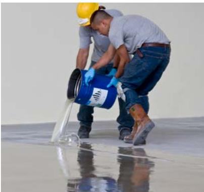
The material is poured onto the floor surface immediately after mixing. The container must be completely emptied.
