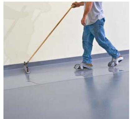
Immediately afterward, this layer must be rolled over with a short-pile epoxy resin-compatible roller in a cross pattern (at 90° angle to the working direction of the squeegee). This ensures that the vapor barrier is evenly distributed on the substrate without any pinholes.
