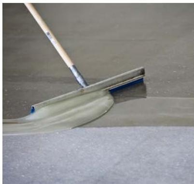
KÖSTER VAP I 2000 systems are applied in one step and distributed with a notched rubber squeegee so that a minimum unbroken layer thickness of 0.4 mm is achieved.
